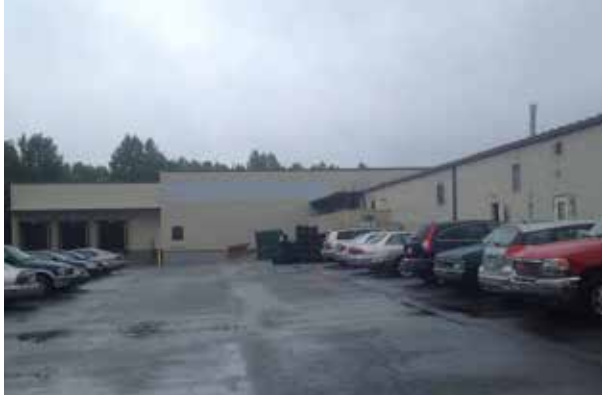
A new addition to expand capacity at Archer Advanced Rubber's production facility.
