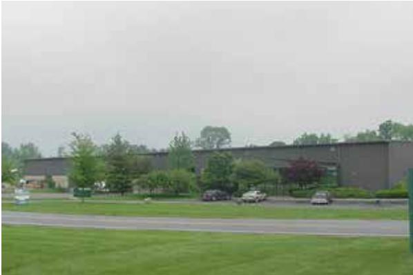
The CAP & Associates headquarters in Columbus, Ohio.
