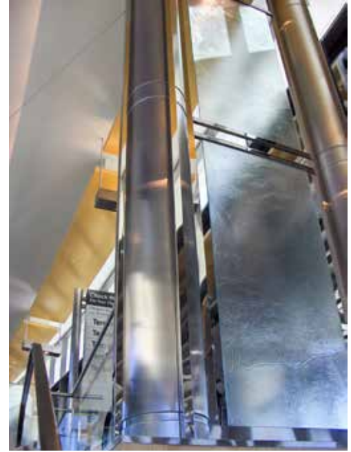
Stainless steel wall cladding for an airport project.
