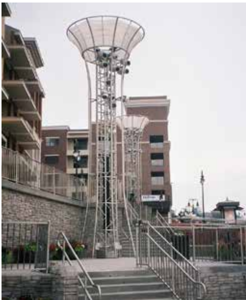
Stainless steel custom light towers for the Branson Landing Shopping Center in Branson, MO.
