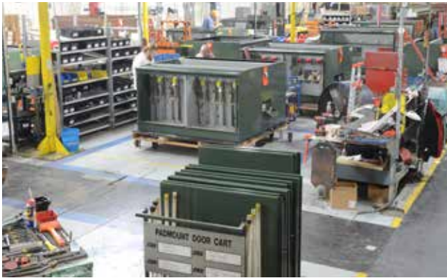
EMC has nearly one million square feet of modern manufacturing facilities located in Virginia, Tennessee and Mexico.
