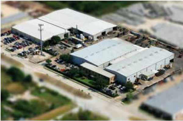
For decades, FabCorp has maintained their sprawling plant facility with the productivity found through ERP software.
