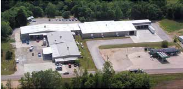
Aerial shot of Hawkeye Industries' facility
