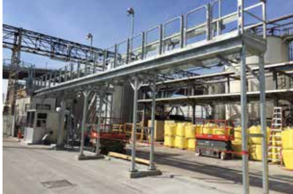
Pictured is Hemco's loading rack, safety gates and SAS gangway.
