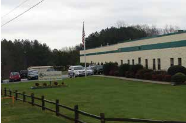
Justrite's 50,000 square foot facility in Anderson, SC.
