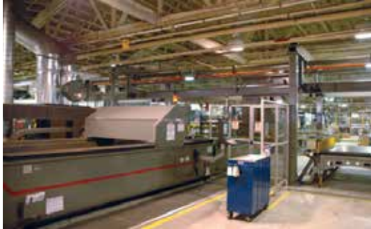
Midland's high-speed laser cell can process 60" x 120" steel sheets up to 7/8" thick.
