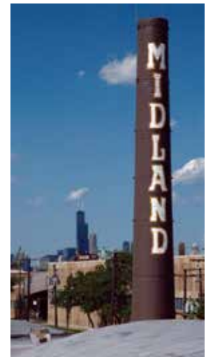
Midland's production plant near the heart of downtown Chicago.
