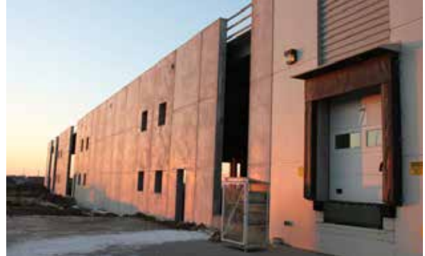
A new addition to PS Garage Doors headquarters.
