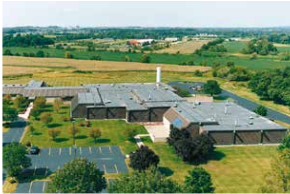
Aerial view of RAM Precision Industries' campus.
