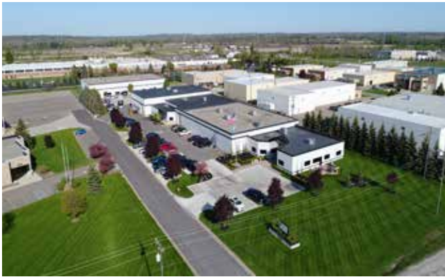
An aerial view of Sharp Tooling Solutions' facility located in Romeo, Michigan.
