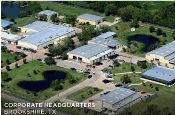
Headquarters for Thomas Instrument in Brookshire, Texas.
